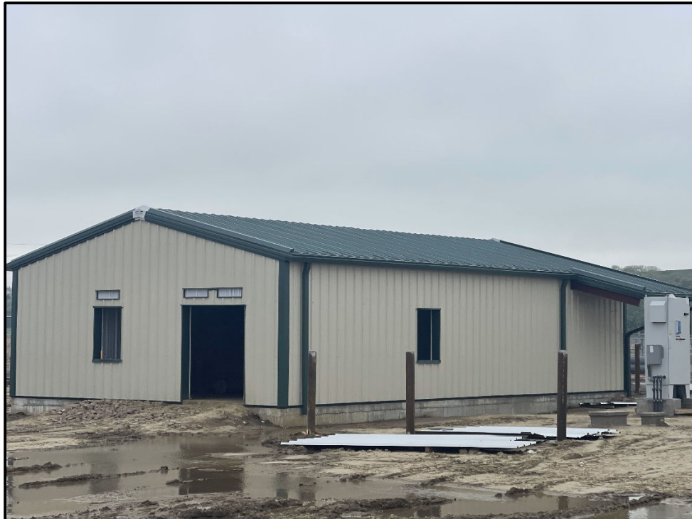
Existing Switchgear Building for Reference
